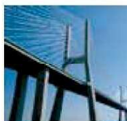
橋梁の振動計測
