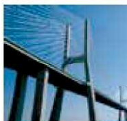
橋梁の振動計測
